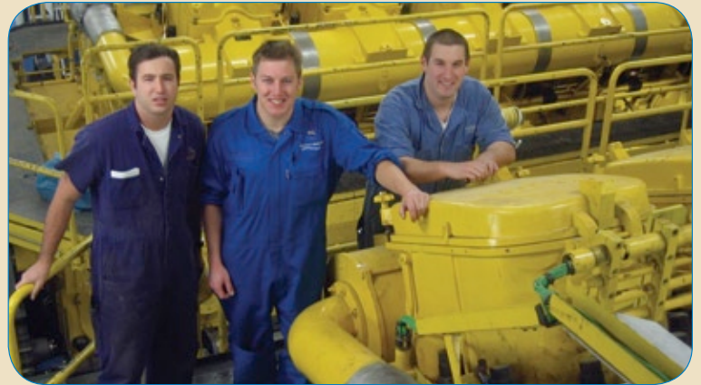
Above: In the ship's engine room are 2nd Engineers Benjamin Young, Adam Vokac and Joe DeMelin all members of the "pride of the Merchant Marine" - the MEBA.
